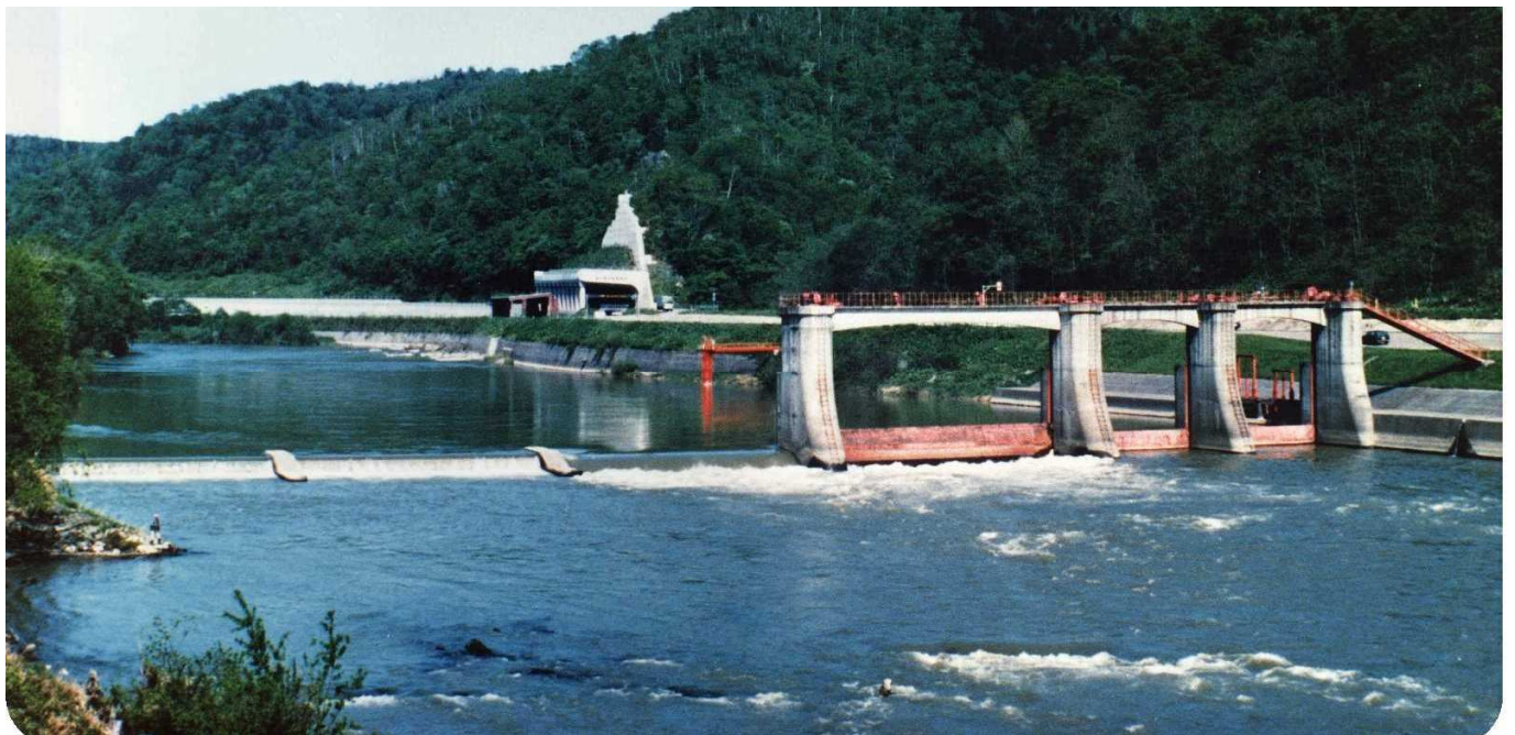
14. Shinryu head works were completed (1961). 2 flushing gates, a spillway, 3 tilting gates and 2 intake gates
